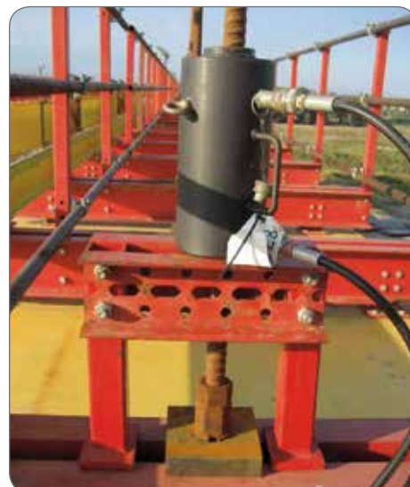
CRI 100/150 FO and CRI 60/250 FO GS cylinders used for lifting structures in the infrastructure sector.
