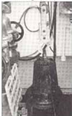
Lifting of submersible sewage pump
