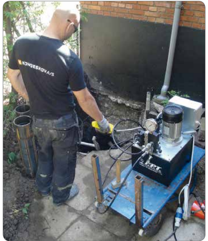
Hydraulic pump with solenoid valve and 20 l tank.
