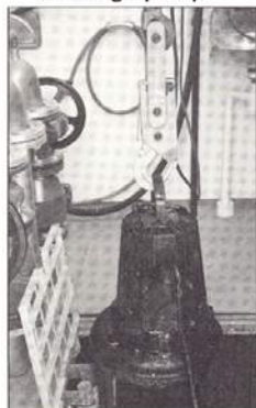
Lifting of submersible sewage pump
