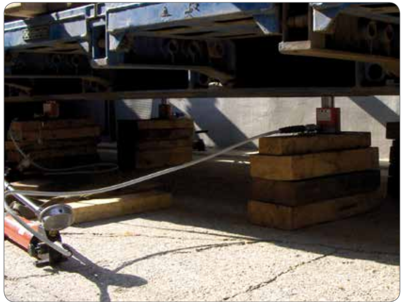
Compact cylinders F.P.T. model - CRM50/50C controlled by two-speed PDSA21 hand pump to level a structure
